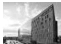
1/ Danube House Karolinská 1 KPF Associates, ADNS Architekti 1998–2003
